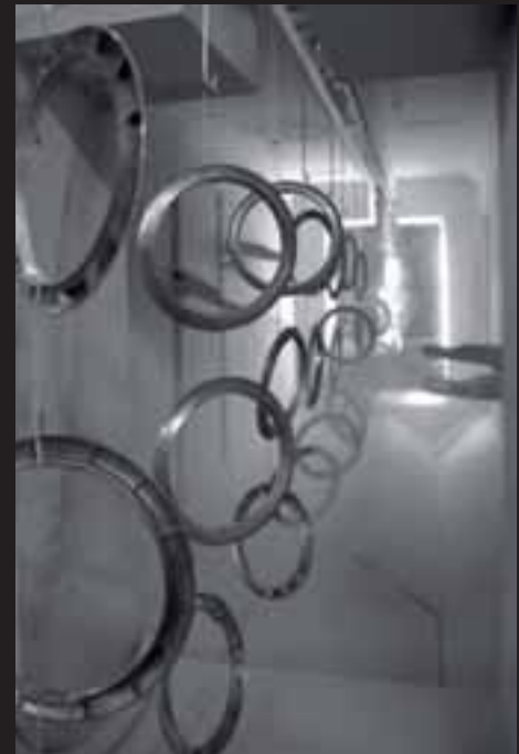
Automatic installation of tunnel for defosfating and degreasing, powder coating booth and polymerization oven.
